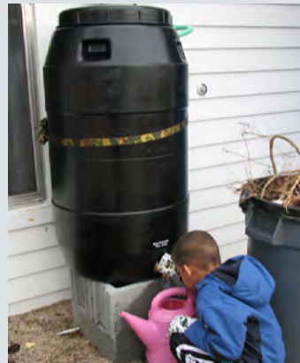
Figure 1. (Left) Elevate barrel and cut downspout
